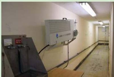
To prevent sanitation issues the moisture content in the air is lowered by passing the air through the Airwatergreen desiccant dehumidifier. The moisture is removed preventing plant damage and potential contamination issues
